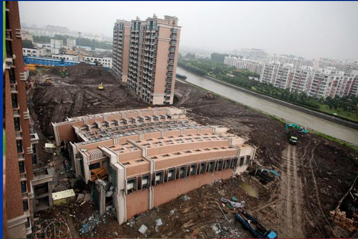
Lotus Riverside Shanghai collapse: Corruption in building codes
